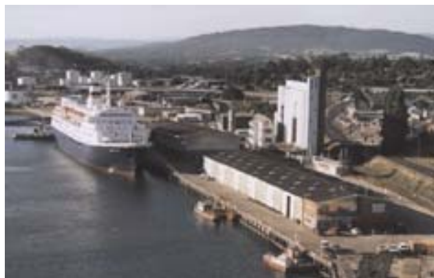
Devonport—No. 3 Berth West and No. 4 Berth West
