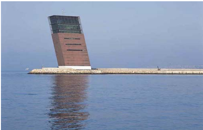
Lisbon Harbor Control Tower
