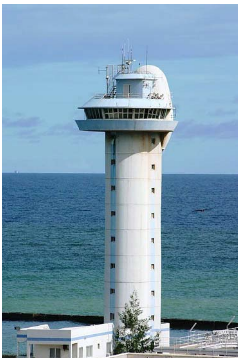
Dakar Harbor Control Tower
