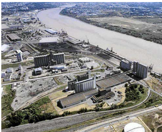
Bordeaux—Dry Bulk and Timber Quay
