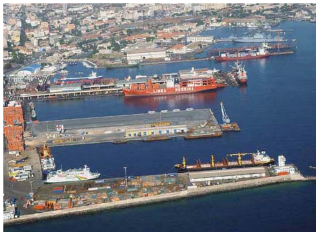
Dakar Port—Southern Zone Piers from E
