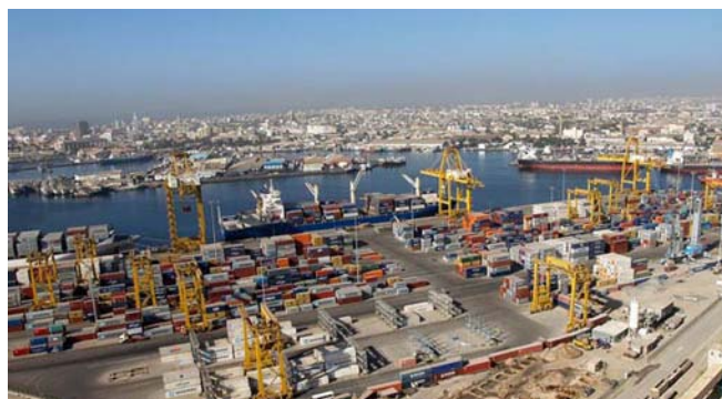
Dakar Port—Container Terminal from NE
