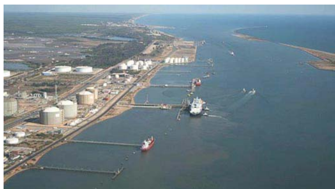
Huelva—Petro Terminal from NW
