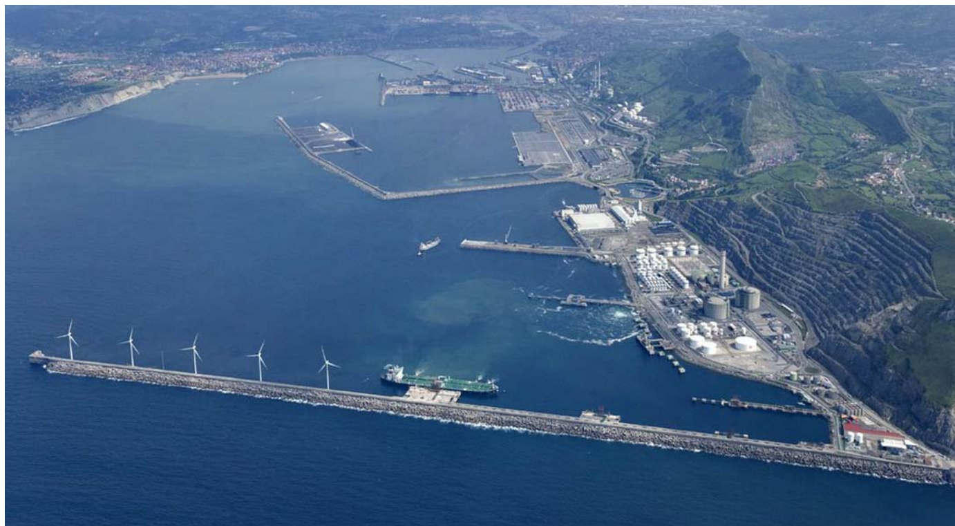
Bilbao—Punta Lucero Breakwater from W
