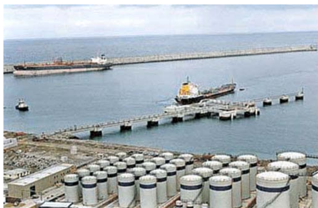
Bilbao—Punta Lucera Breakwater from SE
