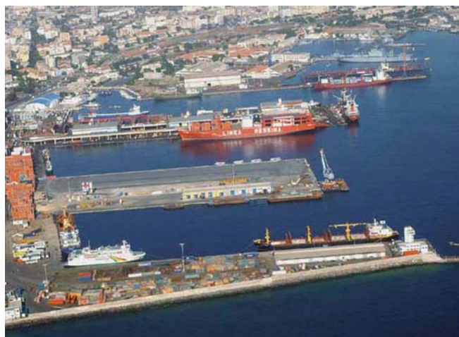
Dakar Port—Southern Zone Piers from E
