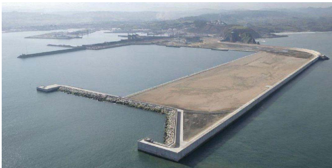
Gijon—Bulk Quay (under construction)
