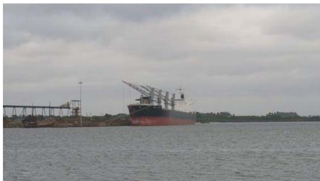
Buchanan Ore Loading Terminal
