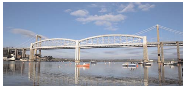
The Royal Albert Bridge and the Tamar Bridge
