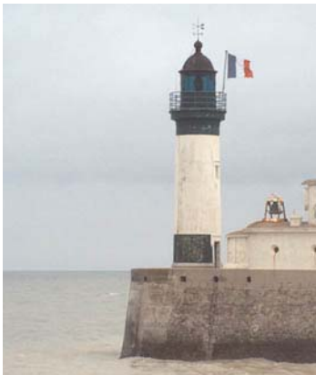
Le Treport Light (West Breakwater)
