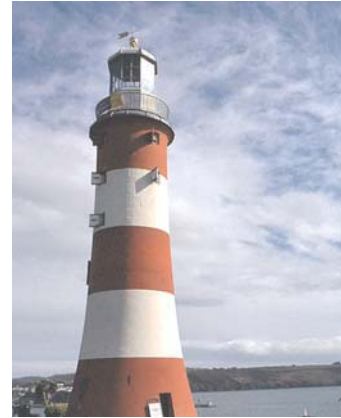
Smeaton Tower (disused)
