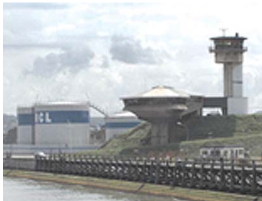
Boulogne Port Control Tower
