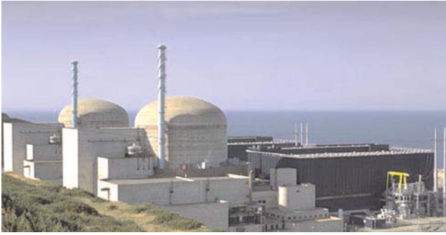
Flamanville Nuclear Power Station
