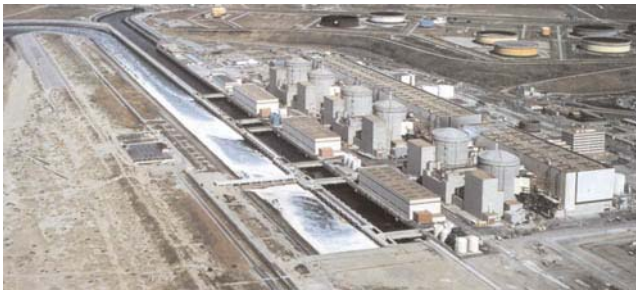
Gravelines Nuclear Power Station
