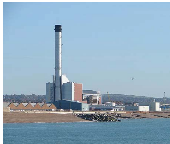
Shoreham Power Station
