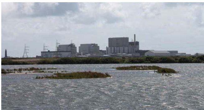
Dungeness Nuclear Power Station
