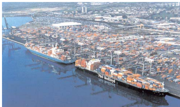
Southampton Container Terminal
