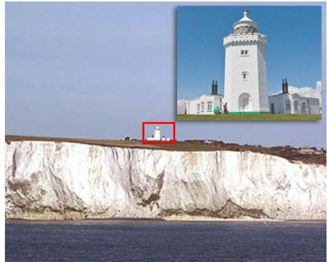
South Foreland Light Tower (disused)
