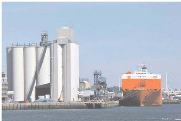
Eastern Docks Silo
