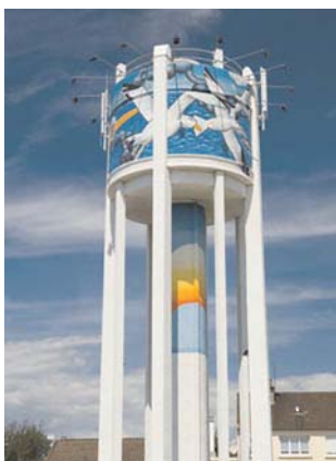
Calais—Bleriot-Plage water tower
