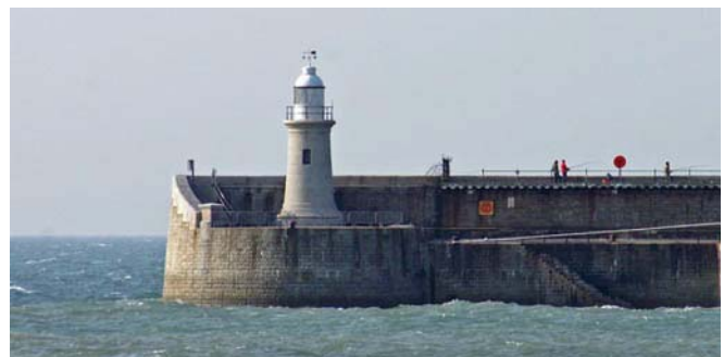
Folkestone breakwater light
